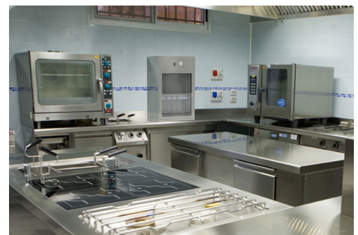
Application in an industrial kitchen
